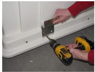
**Step#5** Mark and drill two 3/8" holes as shown. Install two 3/8' x 2.5" hex bolts. Then install from the inside two 3/8' fender washer and two 3/8" nylon lock nuts and tighten.
