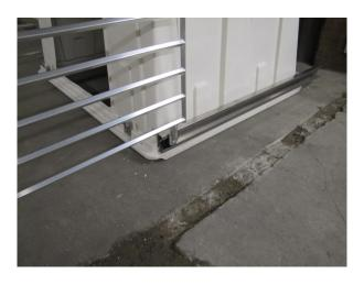
**Step#8** With both side wheels installed on the side gates the next step is to install the front feeding panel
