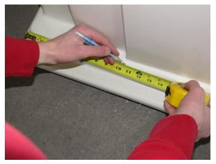
**Step#4** Lock plate installation. There are two lock plates to install. Measure from edge 10.5" as shown above.
